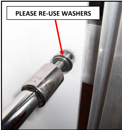
PIC #6: REPLACE EXISTING BOLTS
